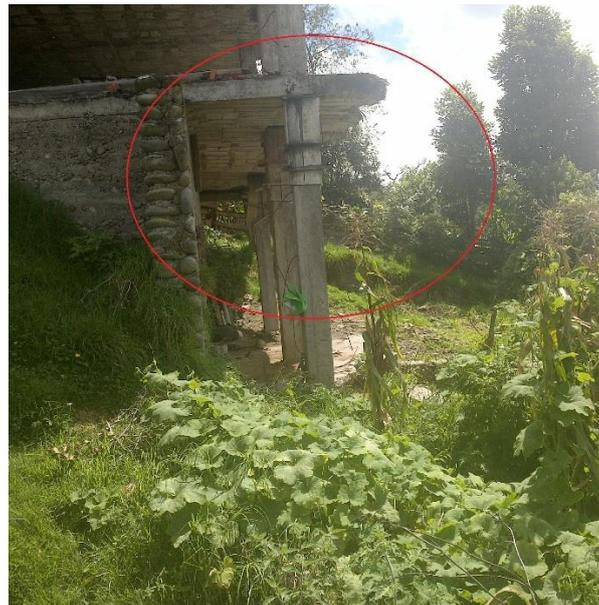
**FOTOGRAFÍA NRO. 35 FRACTURAS QUE INDICAN LA PÉRDIDA DE APOYO EN LA PARTE BAJA, COLUMNAS INCLINADAS A FAVOR DEL DESLIZAMIENTO 724676-9688042 Y 724685-9688075.**
